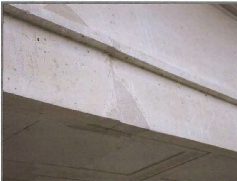
Composite repair on the north-facing portico. Note absence of fractures or separations in the repair.
