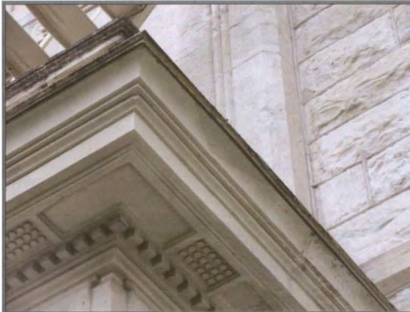
Composite repair on the north-facing portico.
