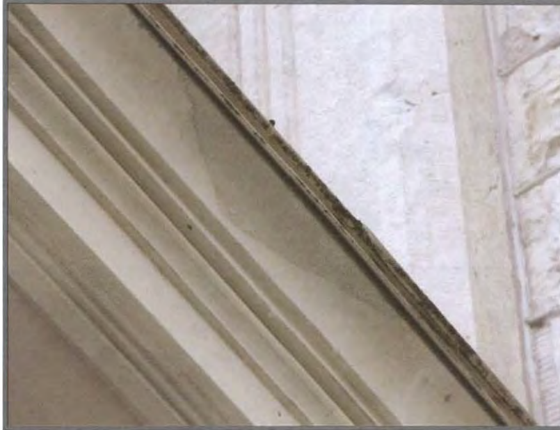
Composite repair on the north-facing portico.
