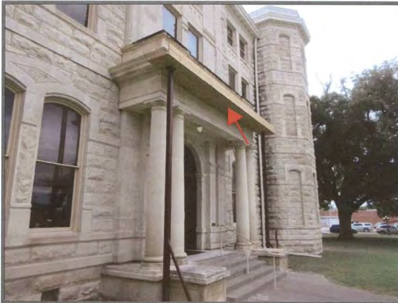
Portico on the west-facing elevation. Note safety structure along the west-facing stone cornice.
