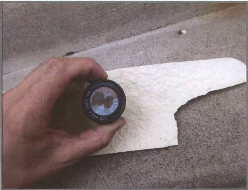
10x magnifier utilized for close observation of the epoxy and drill hole.
