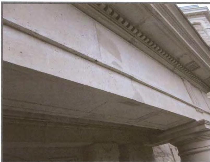
Composite repairs on the north-facing portico.
