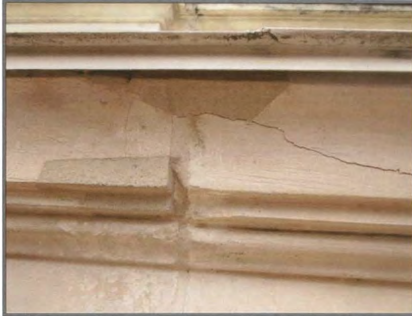
Composite repair on the west-facing portico.
