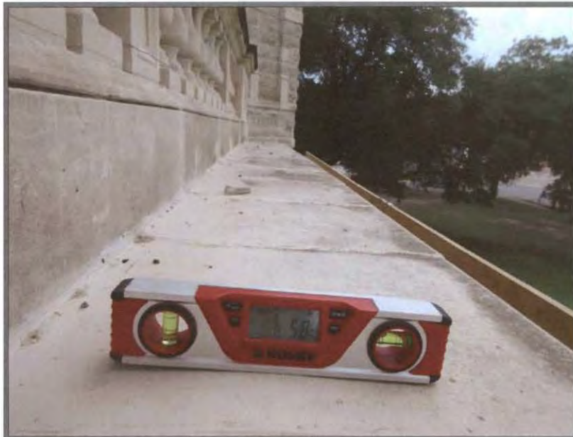
Typical soldered metal panels covering the top of the stone cornice on the porticoes.
