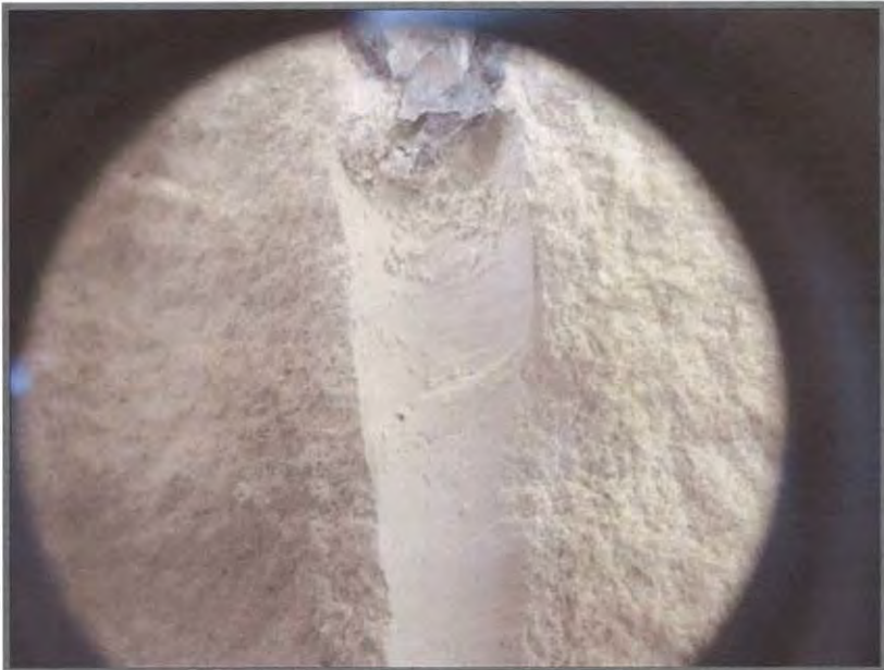
Close-observation of the bottom of the epoxy and drill hole. Note absence of corrosion.
